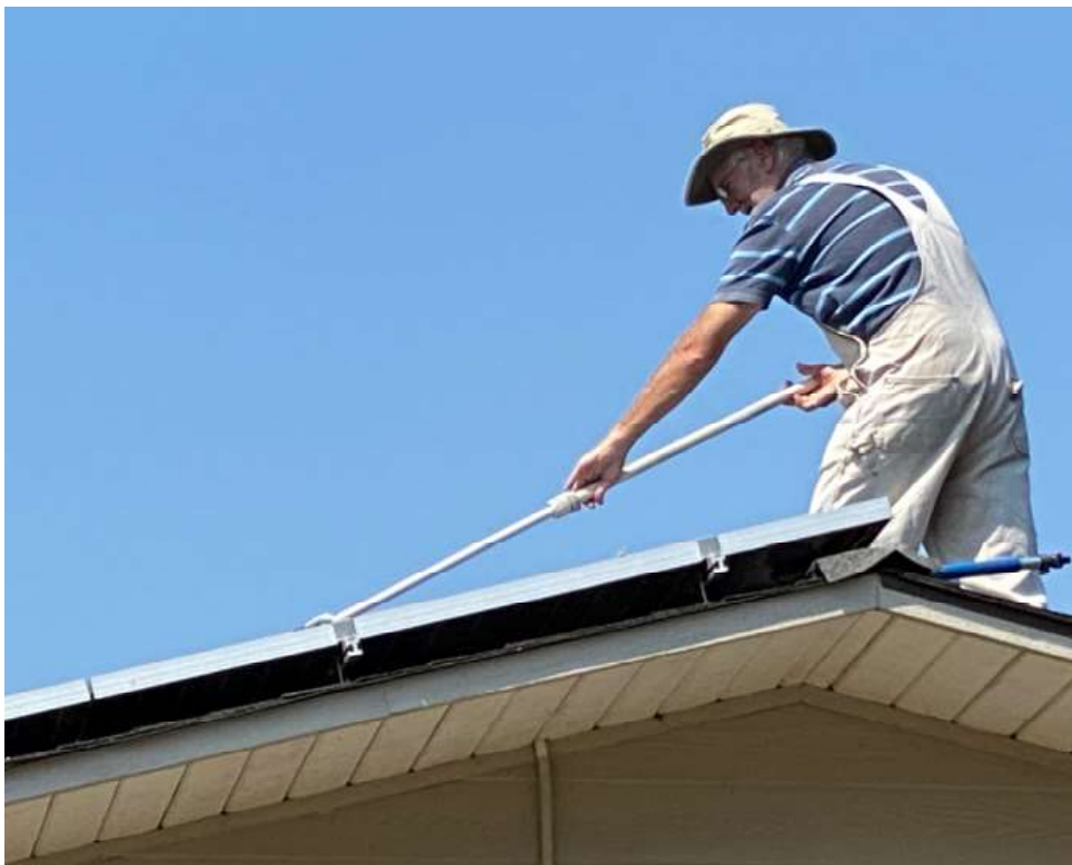
Cleaning the solar array
